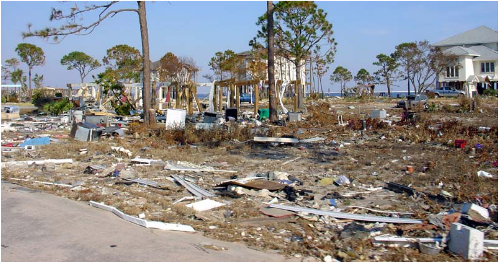
typical hurricane damage
